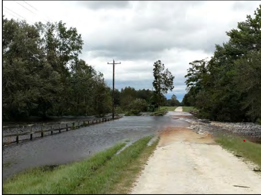
Photos of Camp Branch Creek on Caravelle Ranch Wildlife Management Area immediately after the storm and 1 day after the water receded below road levels. (Photo credit: Jodi Slater)
